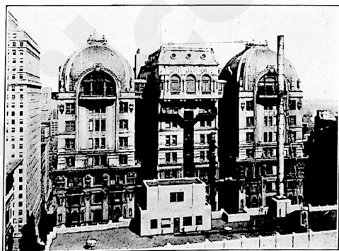
An Installation of the Philco Three Purpose Antenna System on top of a 21-story hotel building. The antenna transformer is mounted on top of the dome at the right, and is grounded to the steel framework of the supporting structure. The transmission line is carried from this point down to the radio set on the thirteenth floor.
