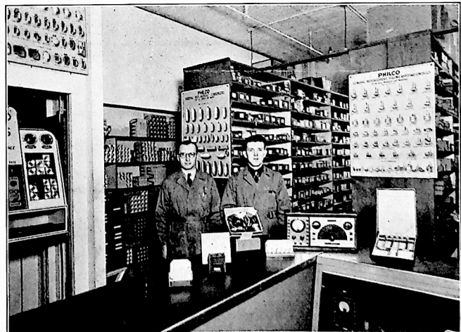
Parts Department, Sunset Electric Company, PHILCO Distributors in Seattle, Wash.
