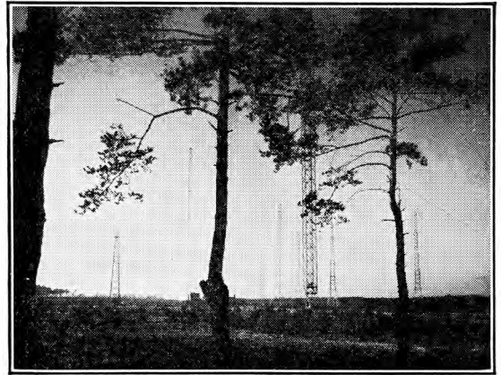
This is an unusually striking photograph of the transmitting antennæ of the powerful German short-wave stations at Zeesen. A complicated system of directional antennæ enable the German programs to be received in America almost daily.
