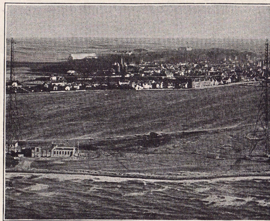
AERIAL VIEW OF KALUNDBORG STATION
