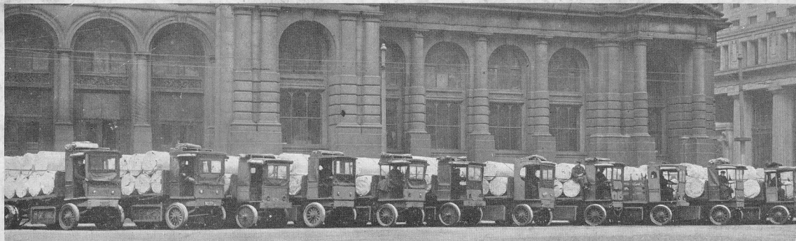
Fleet of Electric Motor Trucks Operated by Blinn, Morrill & Company, Boston
