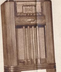
624 P Philco Photo-Electric Reproducer. 7-tube Phonograph Circuit. Tilt-Front Cabinet. Overseas Wave-Band. Built-In Amerseas Wave-Band. Built-In American and Overseas Aerial System. Permanent Magnet Speaker. Self-starting Phonograph Motor. Covers Standard Broadcasts, American and Foreign Short-Wave, State
