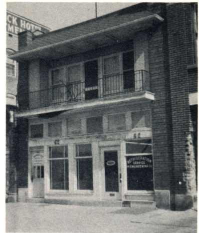
This is the headquarters building of Refrigeration Service & Engineering Co. in Salt Lake City.
