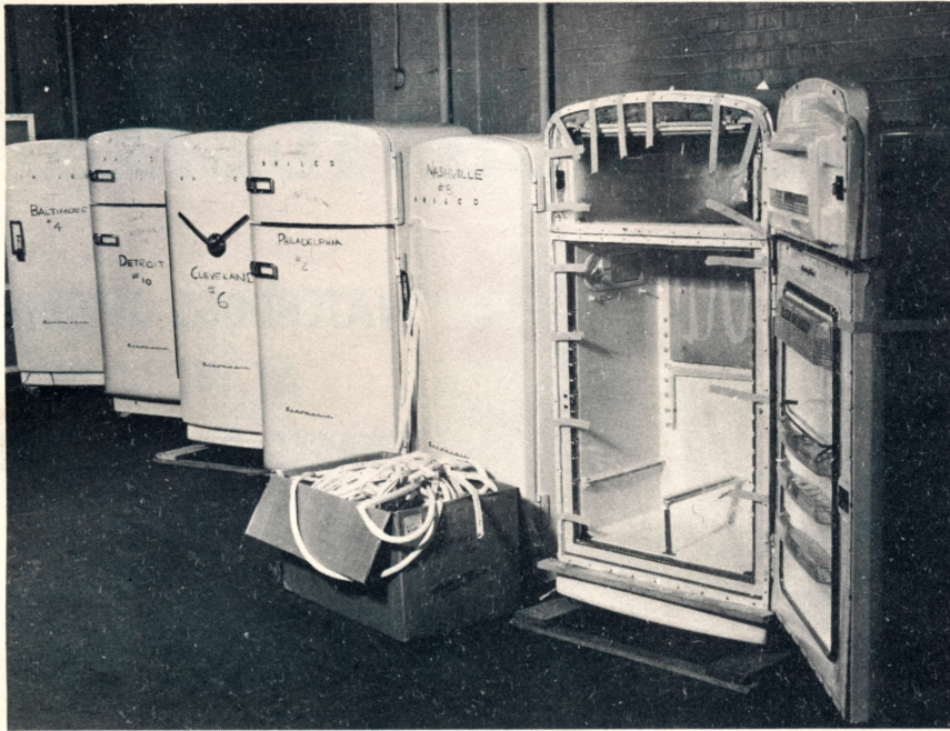
Refrigerators from cities where complaint existed were shipped to Field Engineering headquarters for intensive study.
