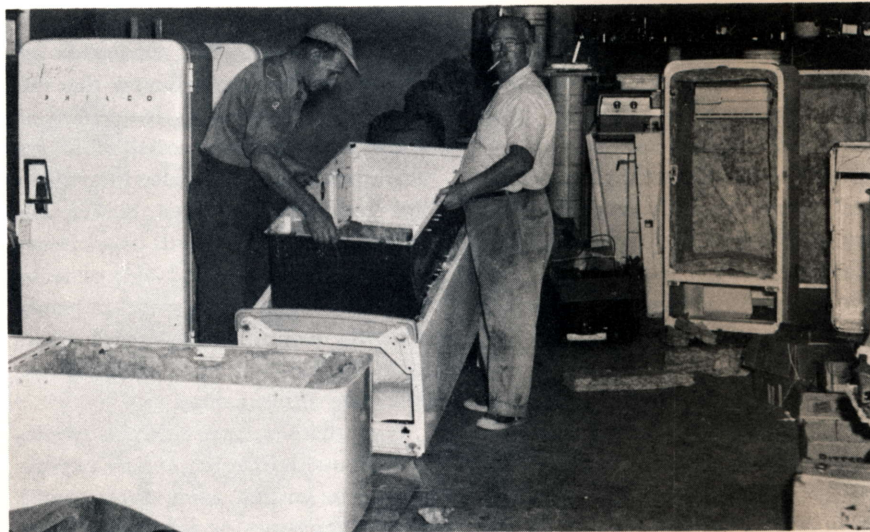
Joe and Frank install a liner in the final stage of reconditioning the appliance. The photographs were taken at Sabatine's, a Philco Dealer in Sandts Eddy, Penna.
