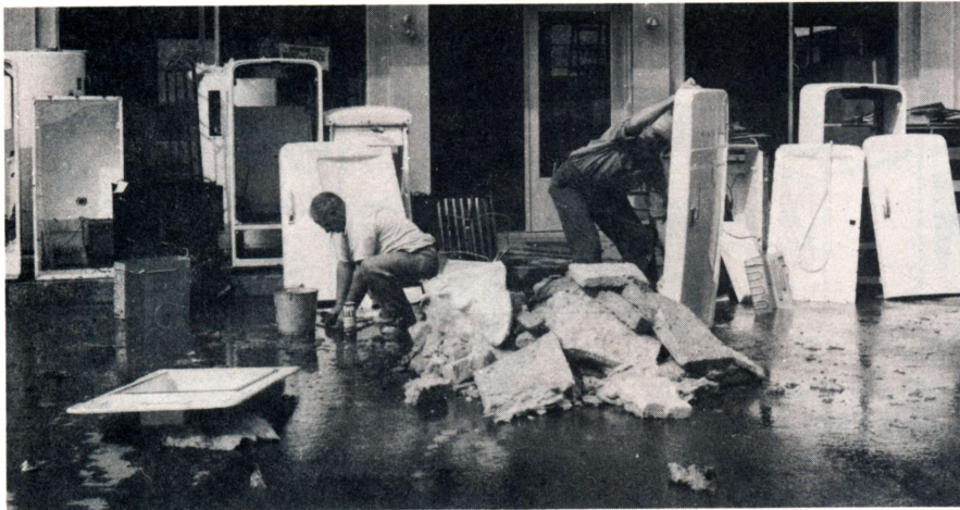
Joe Bean, left, and Frank Tressel, of Philco Service Headquarters, remove damaged insulation and scrub parts before sanitizing appliances.
