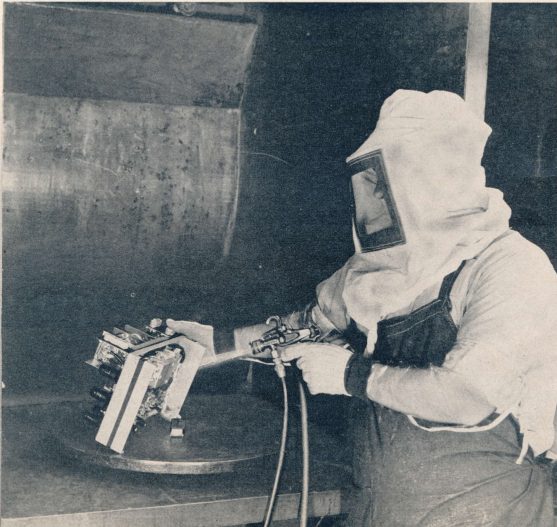
Chemical spraying of radar chassis is part of Philco tropicalization process.
