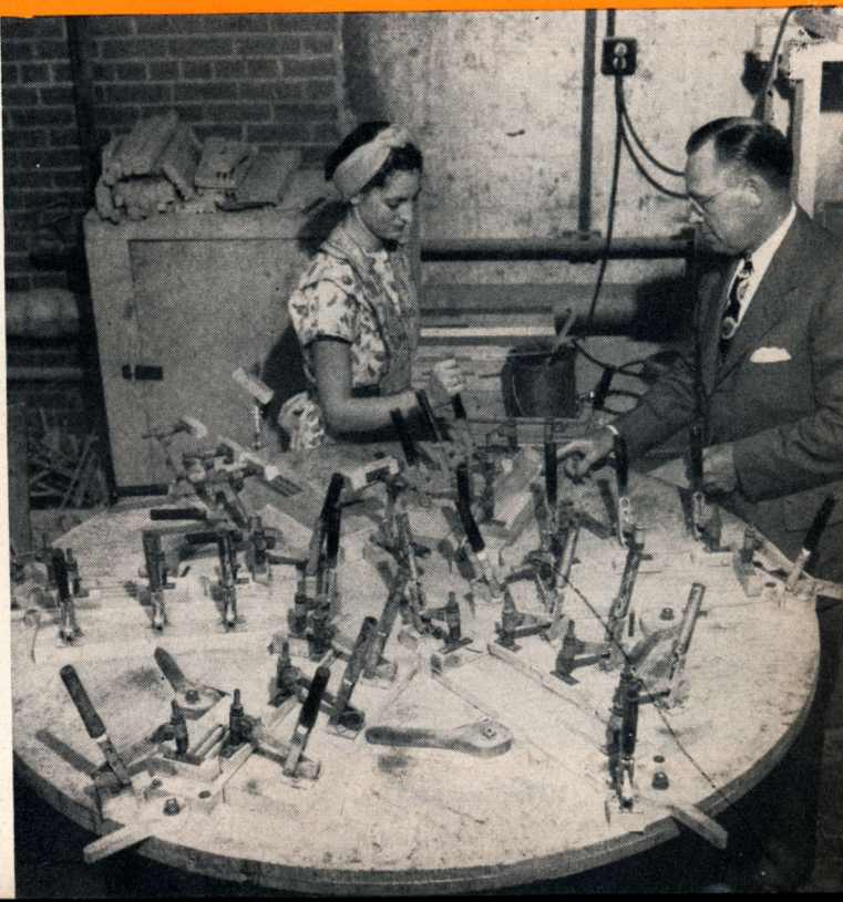
→ Grille overlays and top cleats are glued and then clamped together on this "merry-go-round." As the device revolves, the sub-assemblies dry
