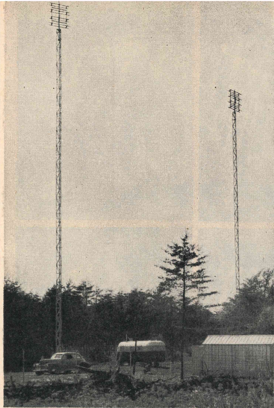
PHILCO'S MULTIPLE-LINK NETWORK BETWEEN WASHINGTON AND PHILADELPHIA
