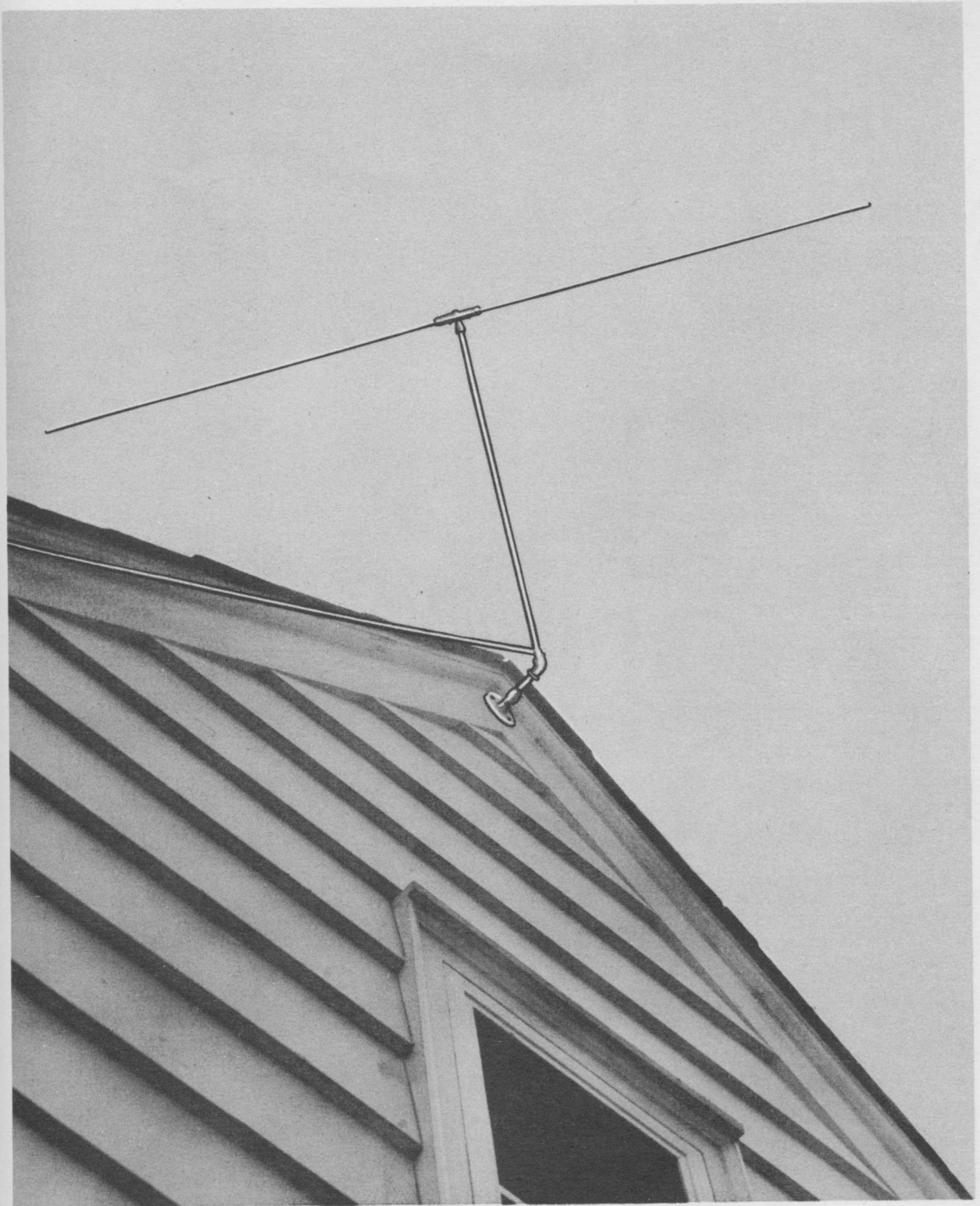
Figure 49C. Single Dipole Antenna Mounted on a Gable.
