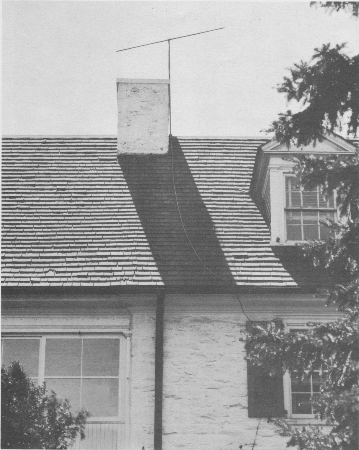
Figure 49B. Single Dipole Antenna Mounted on Ridge of Roof.
