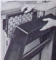
Figure 6. Replacing Air Filter
