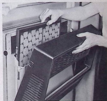
Figure 5. Replacing Air Filter
